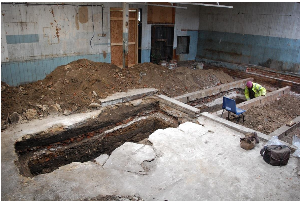
Plate 2. Trench 2 looking north-east.
