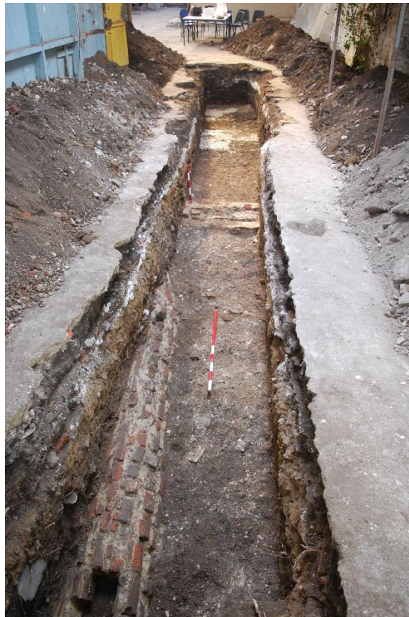
Plate 5. Trench 1. Looking south along the trench, showing brick drain 155 in the foreground, wall 141 running across the trench and chalk floor 177 at the far end. Scales 1m (horizontal) and 0.5m (vertical).
