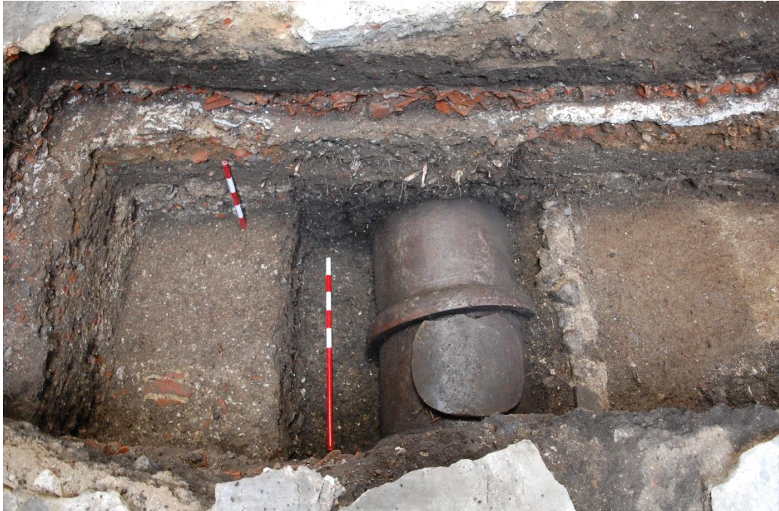
Plate 9. Trench 2. The western side of the western end of the trench, looking north, showing wall 268 and the waste water pipe. Scales 1m (horizontal) and 0.5m (vertical).
