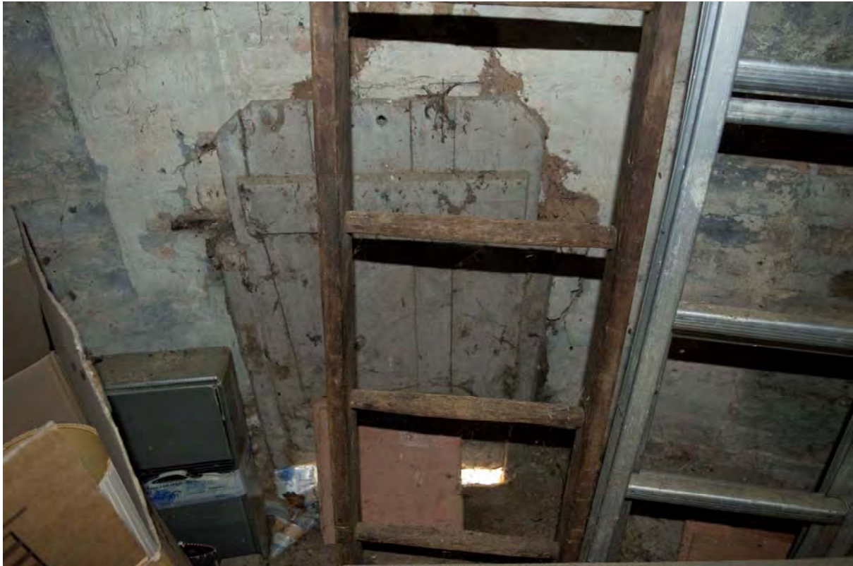
Plate 43 Vertically-sliding timber shutter to the probable stoking hole/fuel door (FMI18-0049)
