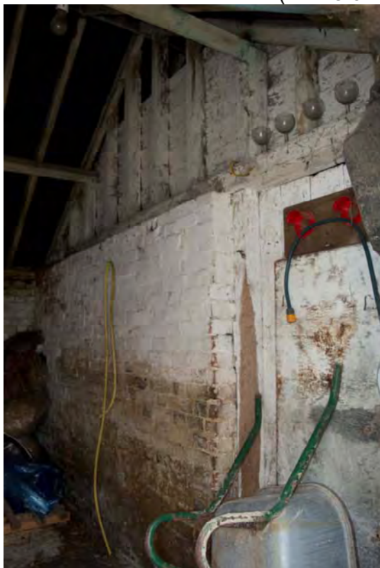
Plate 30 Interior of the stables on the north side of the mill, facing west/north-west, showing the original brick and stud partition between the central and north stables (FMI18-0143)
