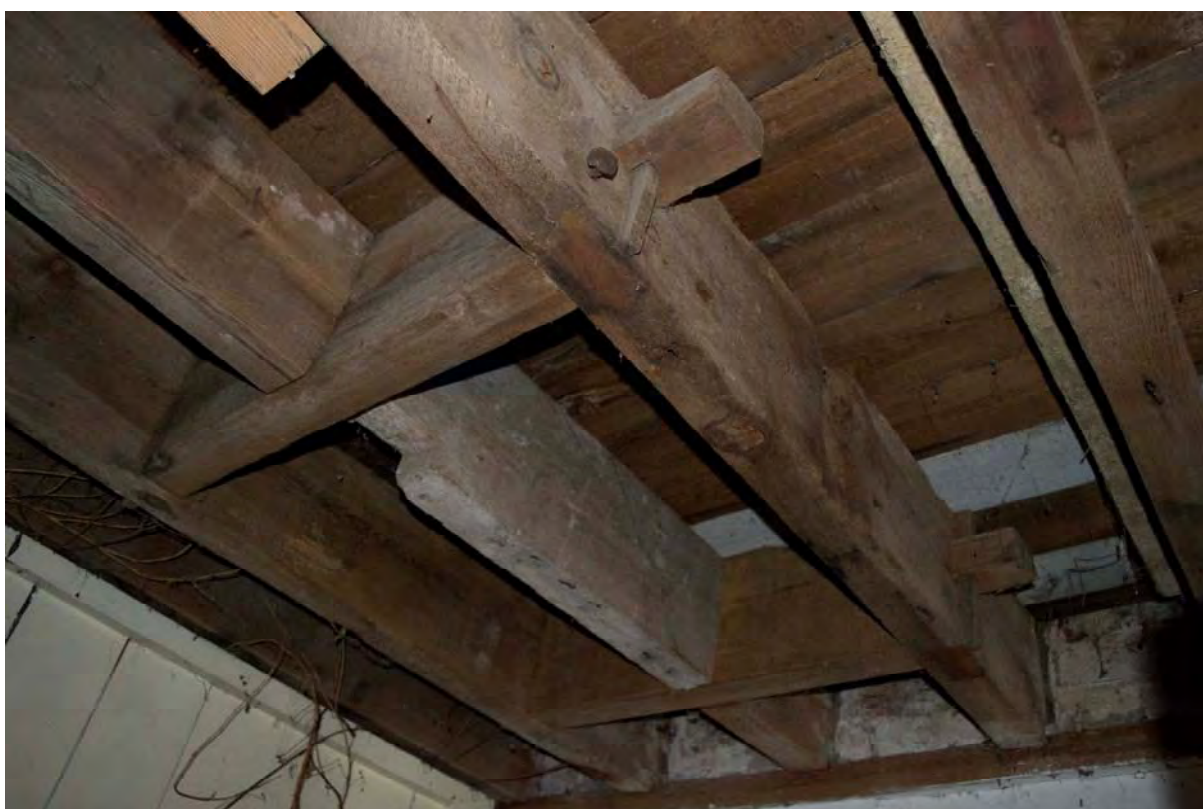
Plate 40 Hatch for probable treading hole (FMI18-0055)
