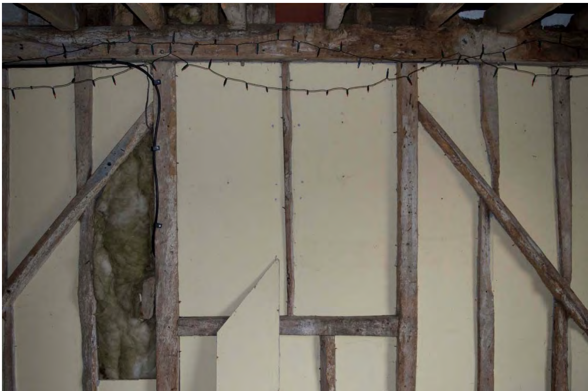
Plate 18 Blocked first floor window within north wall (FMI18-0097)
