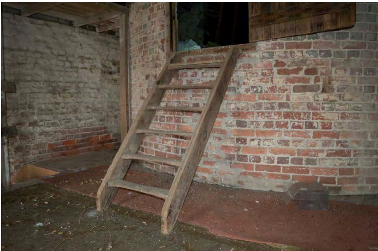
Plate 50 The ladder stair to the drying floor of the roundel (FMI18-0037)
