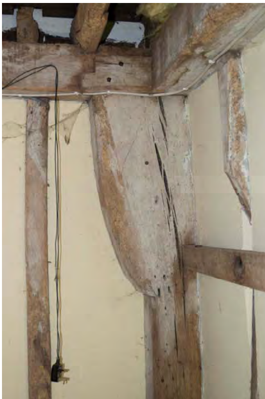
Plate 16 Detail of one of the jowled posts (FMI18-0098)
