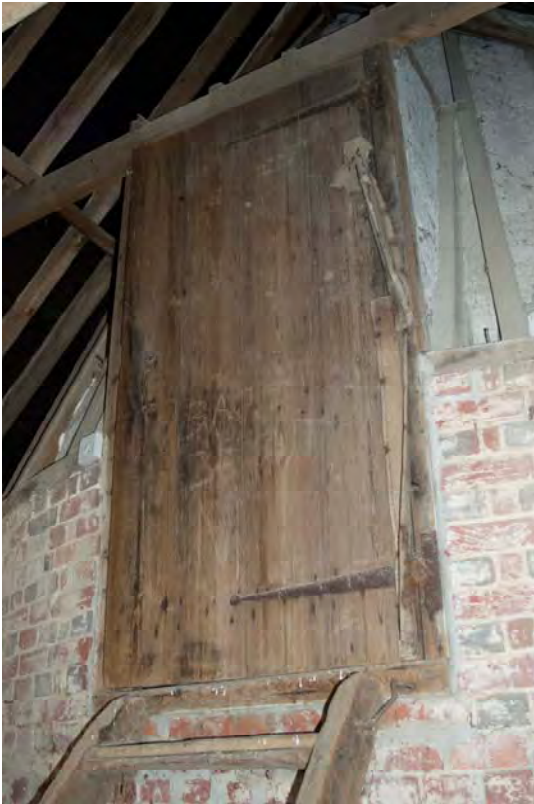
Plate 51 The first floor door to the roundel (FMI18-0038)
