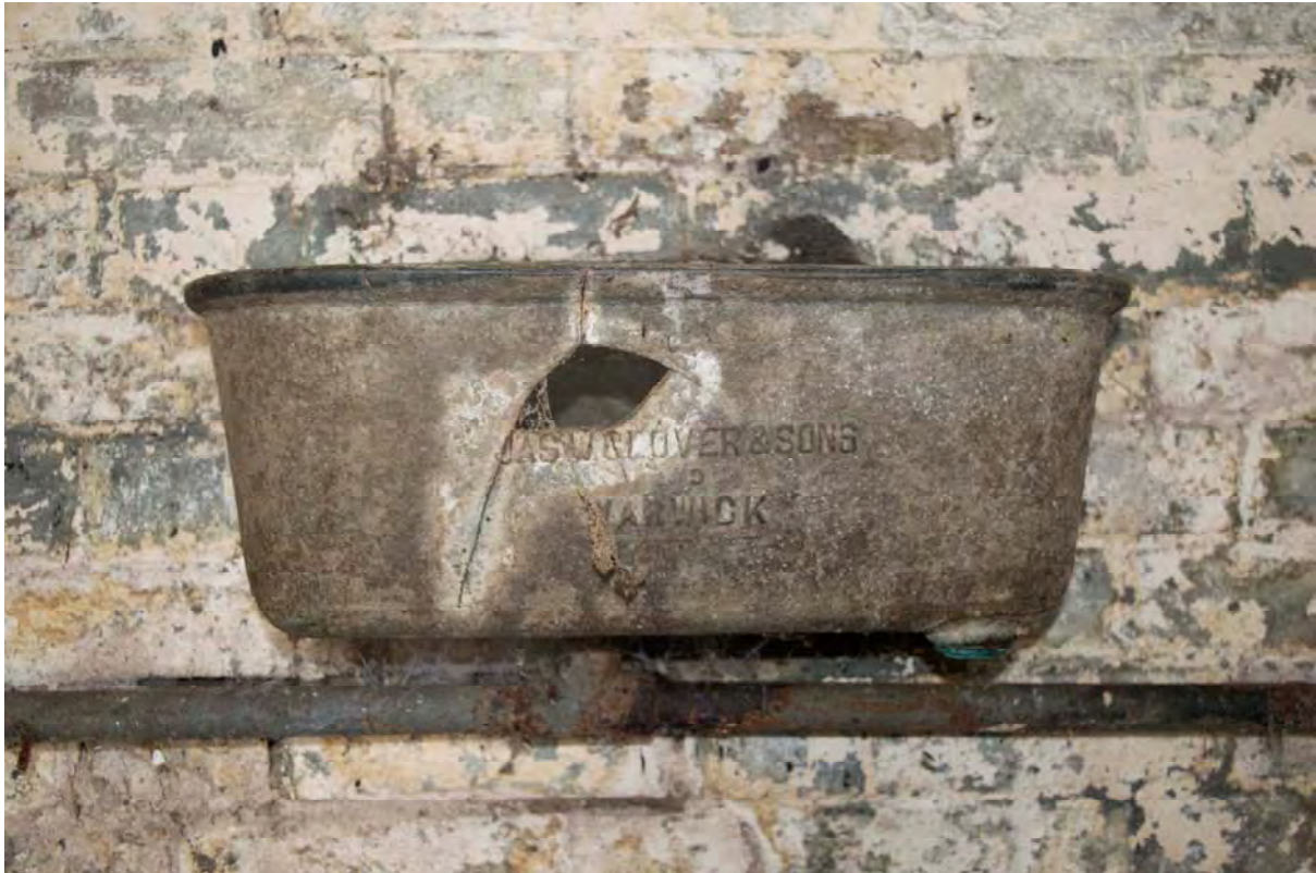
Plate 31 Detail of the water trough on the western wall of the north stable (FMI18-0146)
