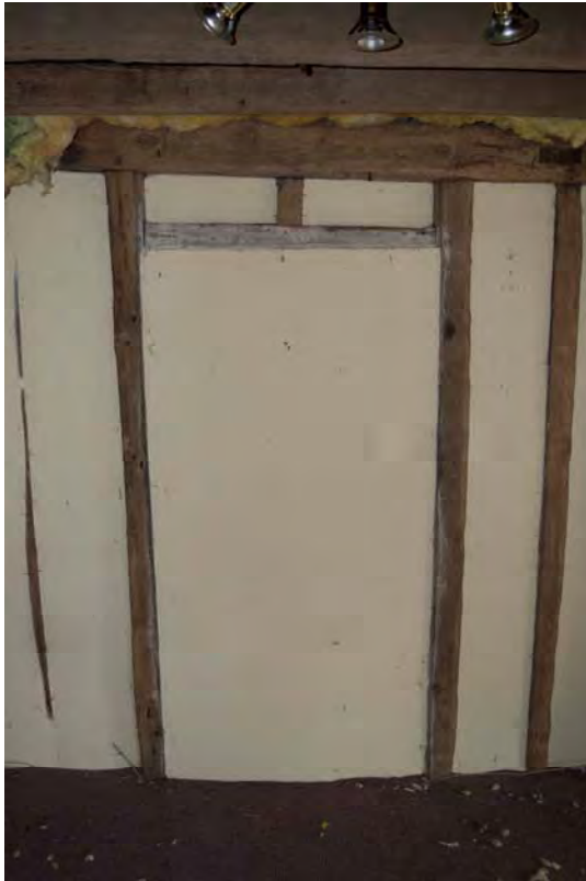
Plate 19 Blocked first floor loading door within east wall (FMI18-0094)
