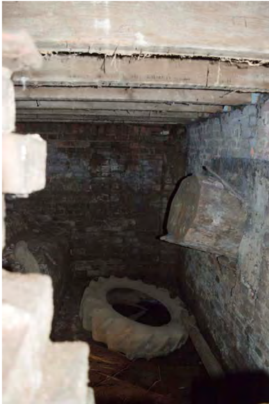
Plate 11 View of the wheelshaft and inserted timber floor, viewed from the passage along the western side of the hurst (FMI18-0123)
