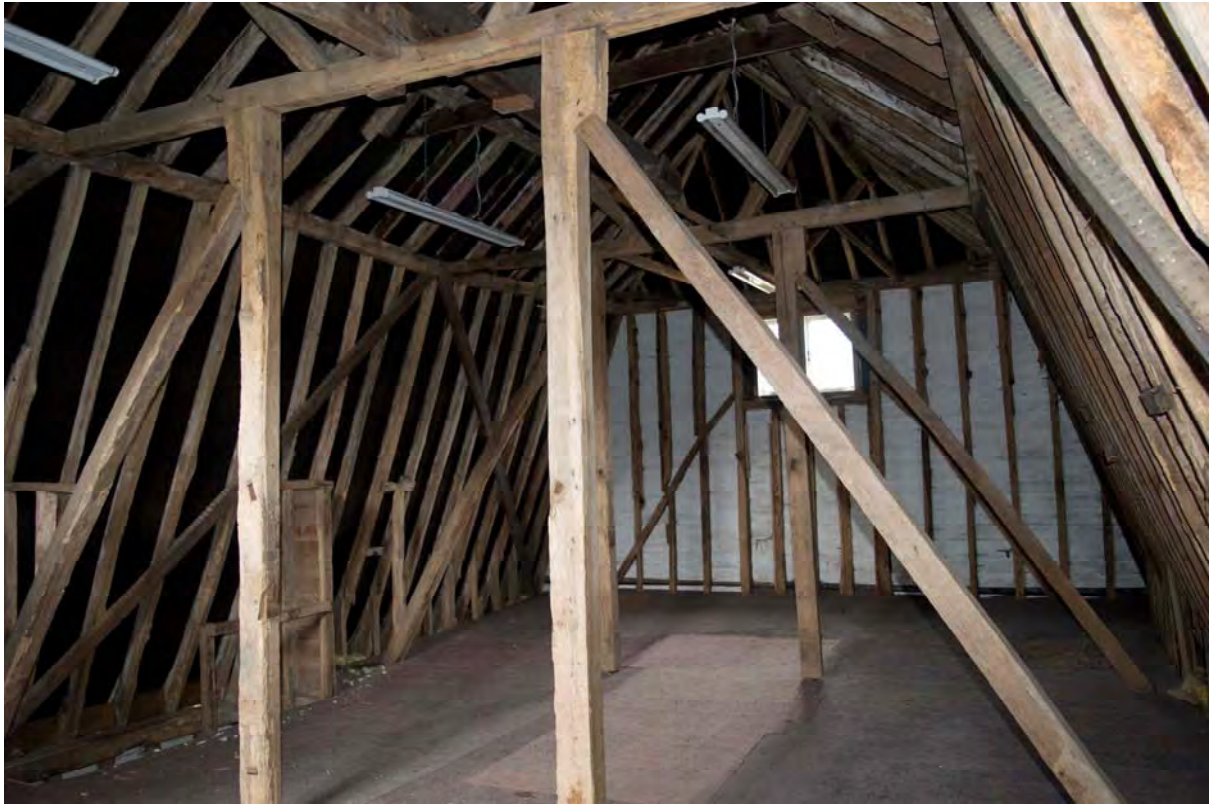
Plate 23 The roof structure/second floor, facing north-west (FMI18-0057)
