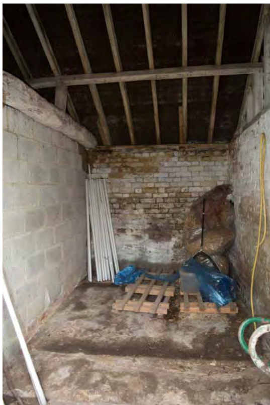
Plate 29 Interior of the stables on the north side of the mill, facing west, showing inserted breezeblock partition between the central and southern stables. Note the drainage channel in the floor (FMI18-0142)
