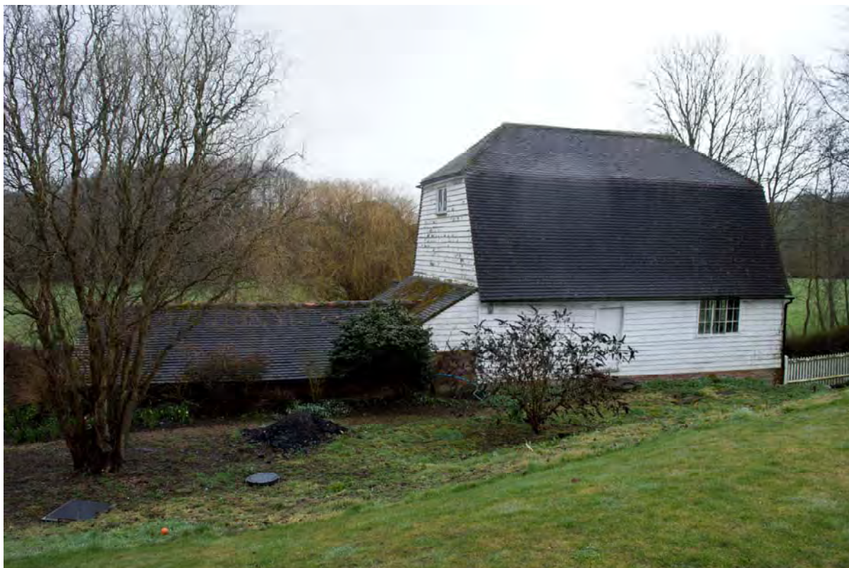
Plate 7 The mill and the mid-19 th century additions, facing east (FMI18-0005)
