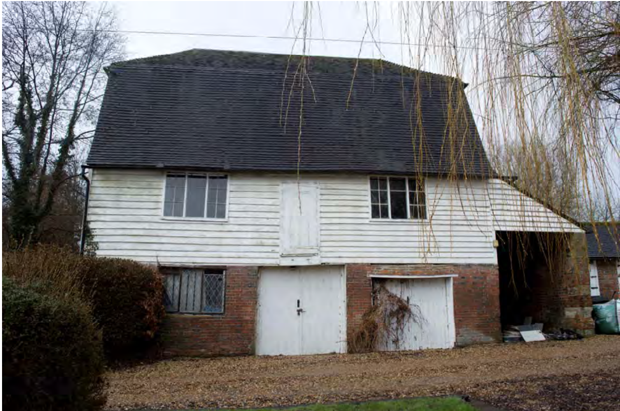
Plate 1 The principal east-facing elevation of the mill (FMI18-0002)
