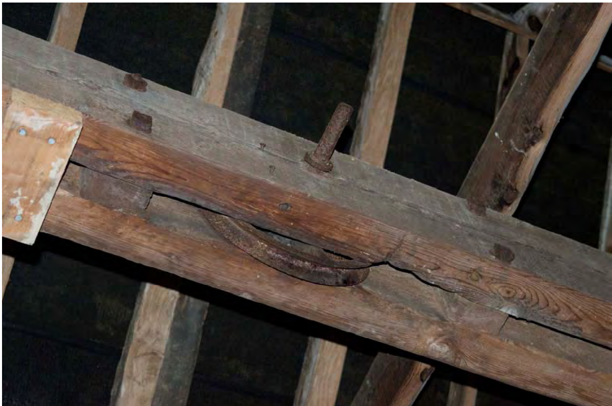
Plate 26 Iron wheel for the sack hoist (FMI18-0124)
