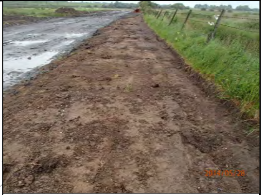
Monks wall pre-construction in the region of trench 3
