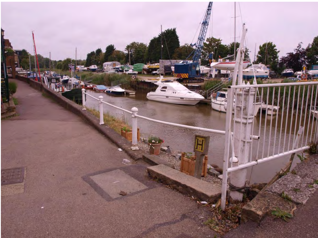
Plate 10: Bollards and water pump located to the west side of the bridge (Bollard No. 1 to left-hand side)
