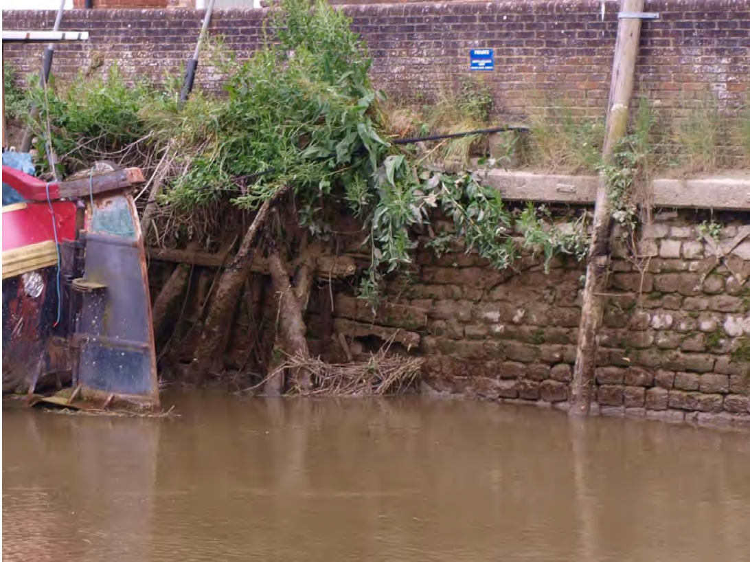
Plate 3: View showing the timber structure overlying the earlier stone walling
