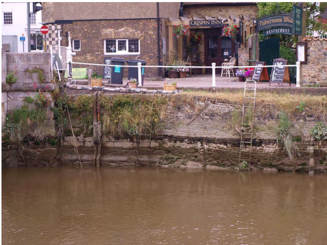
Plate 8: Stonework to the west of the bridge
