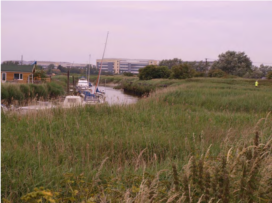
Plate 17: Wharf structure viewed from footpath
