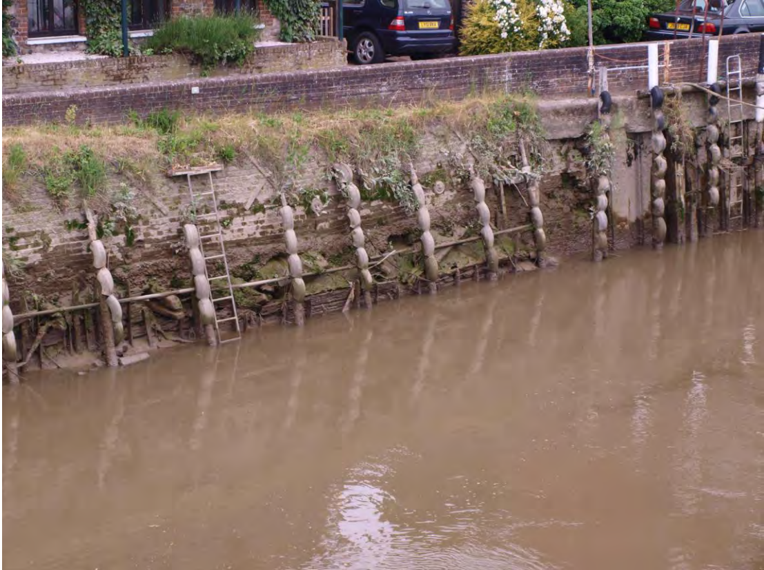
Plate 9: Timber revetment visible at low tide
