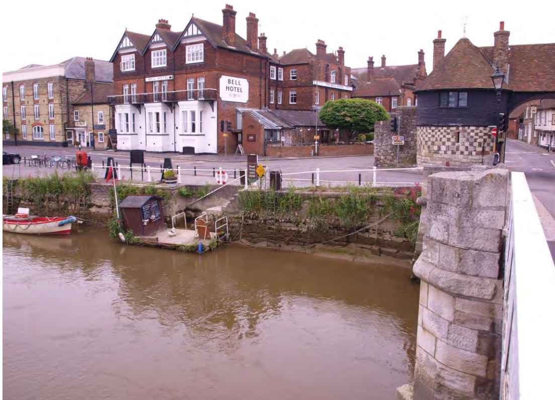
Plate 12: Bollards located to the east side of the bridge (Bollard No. 13 located to right-hand side)
