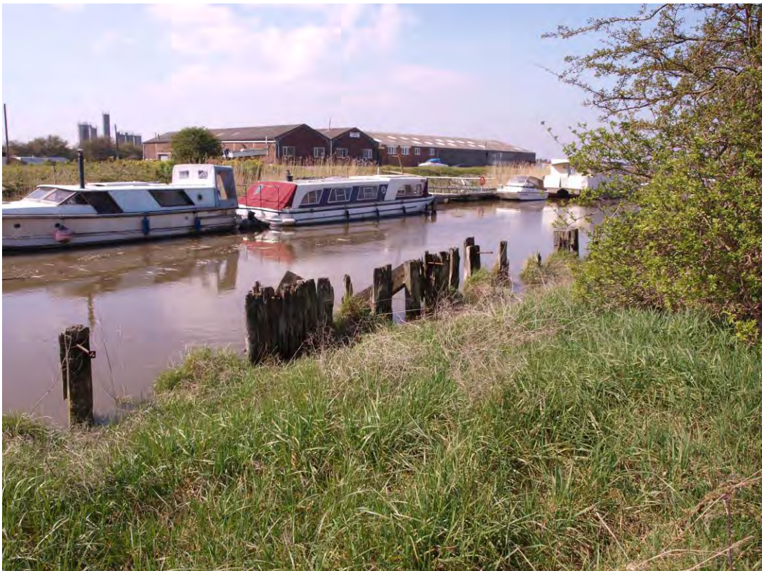
Plate 16: Upstanding wharf structure as viewed from the site
