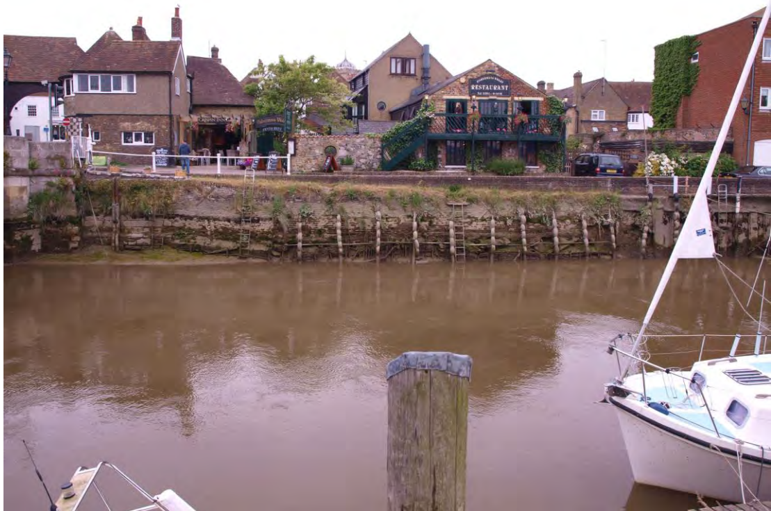
Plate 7: Section 2 of the river wall, showing extent of recorded area
