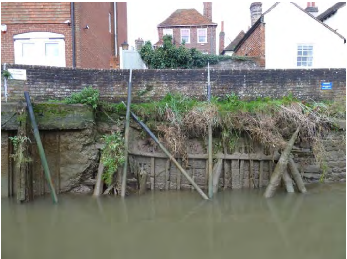
Plate 2: Timber-revetted section of wall to the rear of No. 30
