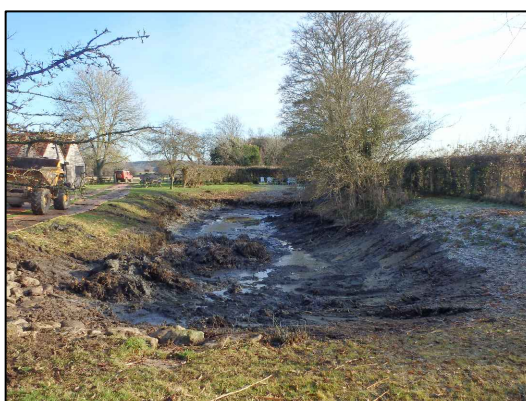
Pond after, looking east
