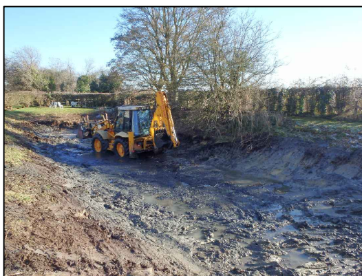
Pond after, looking south east
