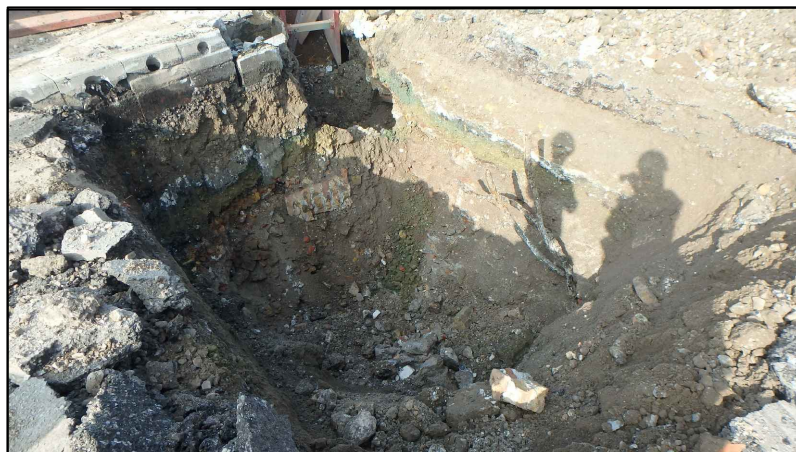
Section facing east, looking north
