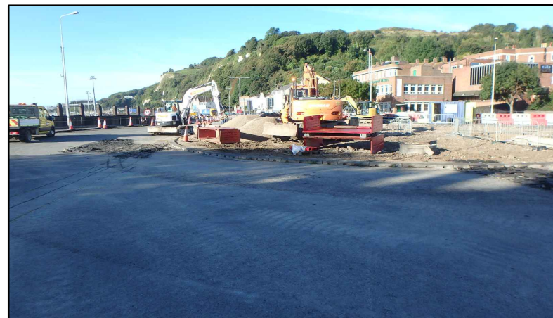
Ground works, looking north west
