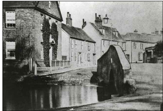
Photo of the 1872 bridge, taken c. 1899
