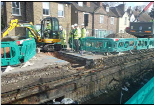
Partially dismantled existing bridge , looking north-east
