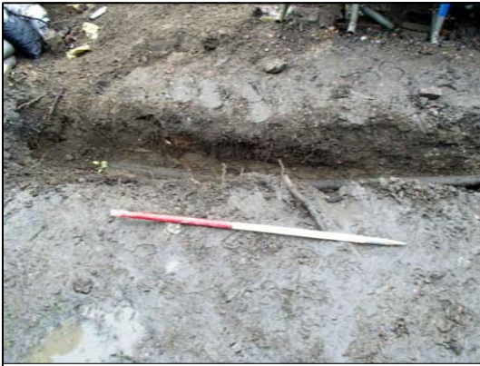
Cable trench excavation
