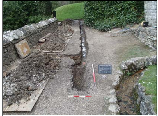
Monitored drainage trench looking north
