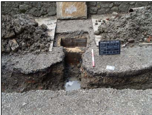
Drainage trench and soakaway looking west
