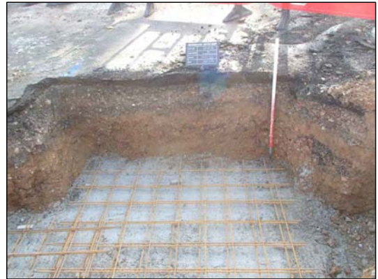
Section 4: southern extent of foundation trench
