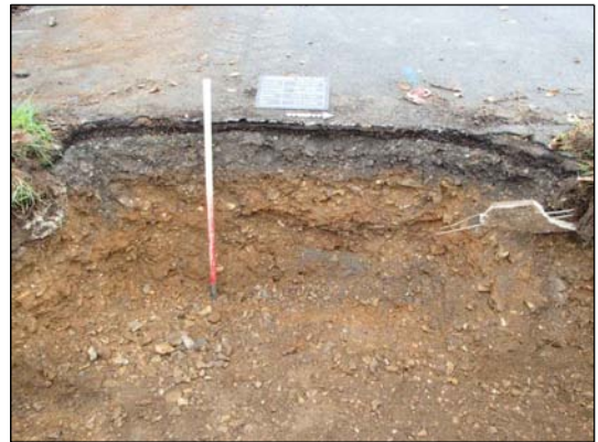
Section 2: eastern foundation trench (facing west)
