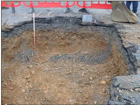
Section 3: eastern foundation trench (facing south)
