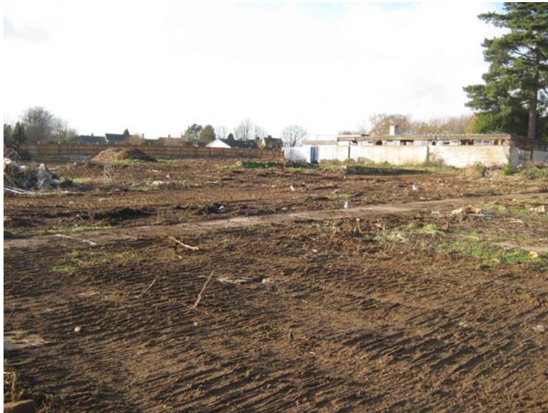
The site, post excavation
