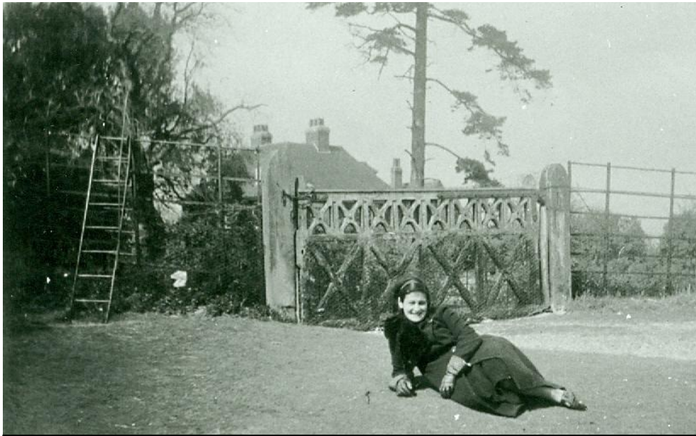
(a) A substantial Victorian wooden park gate, which might have been based on earlier gates at the Park Gate entrance to Lullingstone(55) park. Mildred Reeves c.1930 was the daughter of the then deer keeper. The mild steel park pale dates to the 1890s as does the ladder stile giving public access along a feeder track to the Pilgrim's Way along the south foothills of the North Downs.
