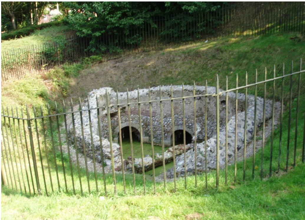
(b) The remains of the conduit house, this structure dating from the seventeenth century, but perhaps on the site of a medieval conduit house. 18 September 2009
