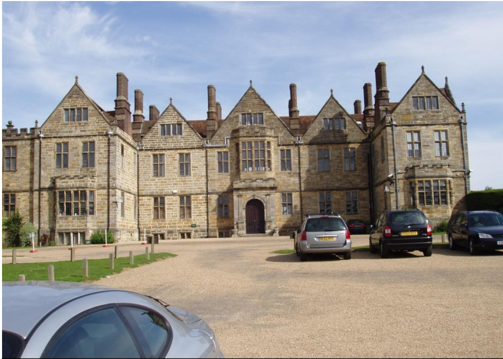
(a) Front elevation of the Jacobean Somerhill mansion, built for the Earl of Clanricarde. 9 September 2006
