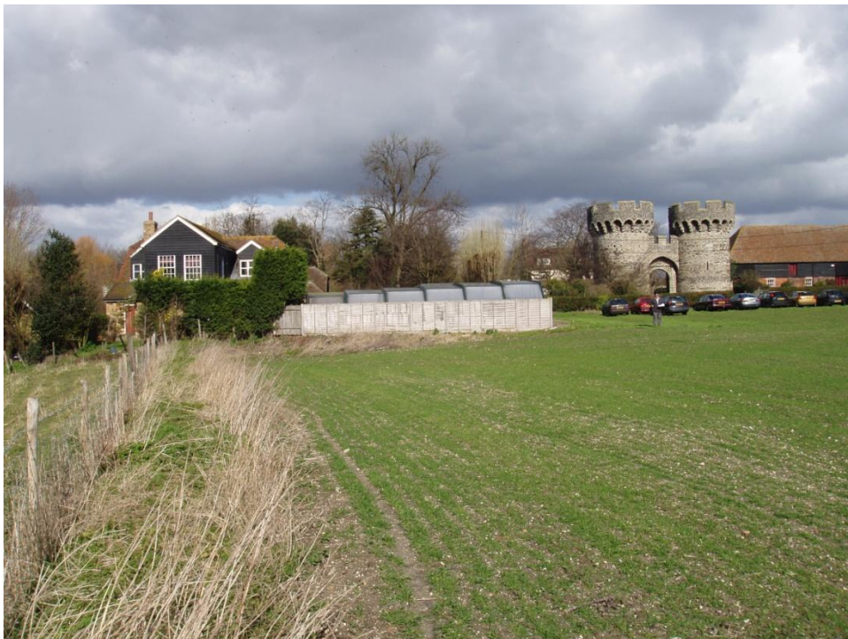
b) South side of Cooling Castle gatehouse. The castle itself overlooks the north Kent marshes. The flat farmland was once part of the park, the west boundary being the bank with fence on the left. 7 March 2007
