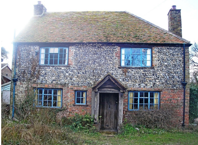
The Cottage before restoration.
