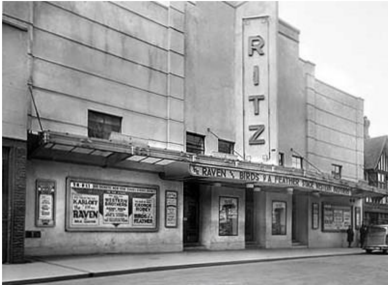
The 'Ritz' cinema in Pudding Lane
