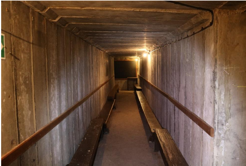
Internal view of the MGS shelter
