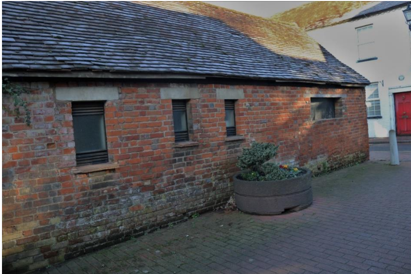
One of the 'Defended Buildings' at Aylesford. The embrasure on the far right was for a 2-pdr A-T gun
