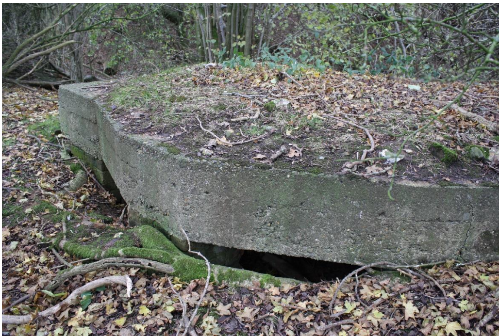
Frontal view showing the firing bays
