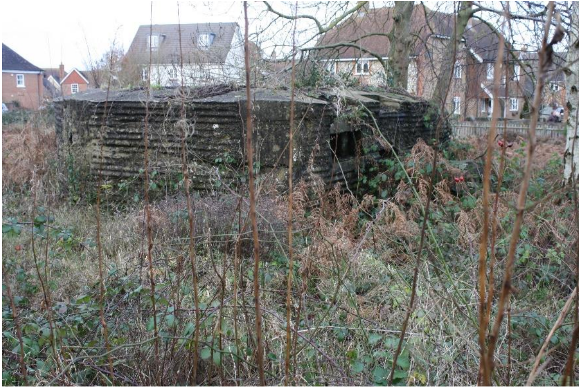
The added concrete strengthening panels can clearly be seen here
