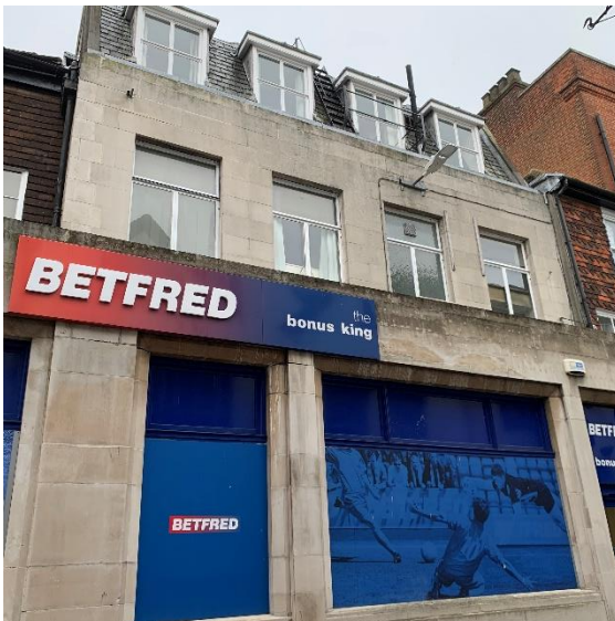
The former General Accident Assurance Company building in Bank Street
