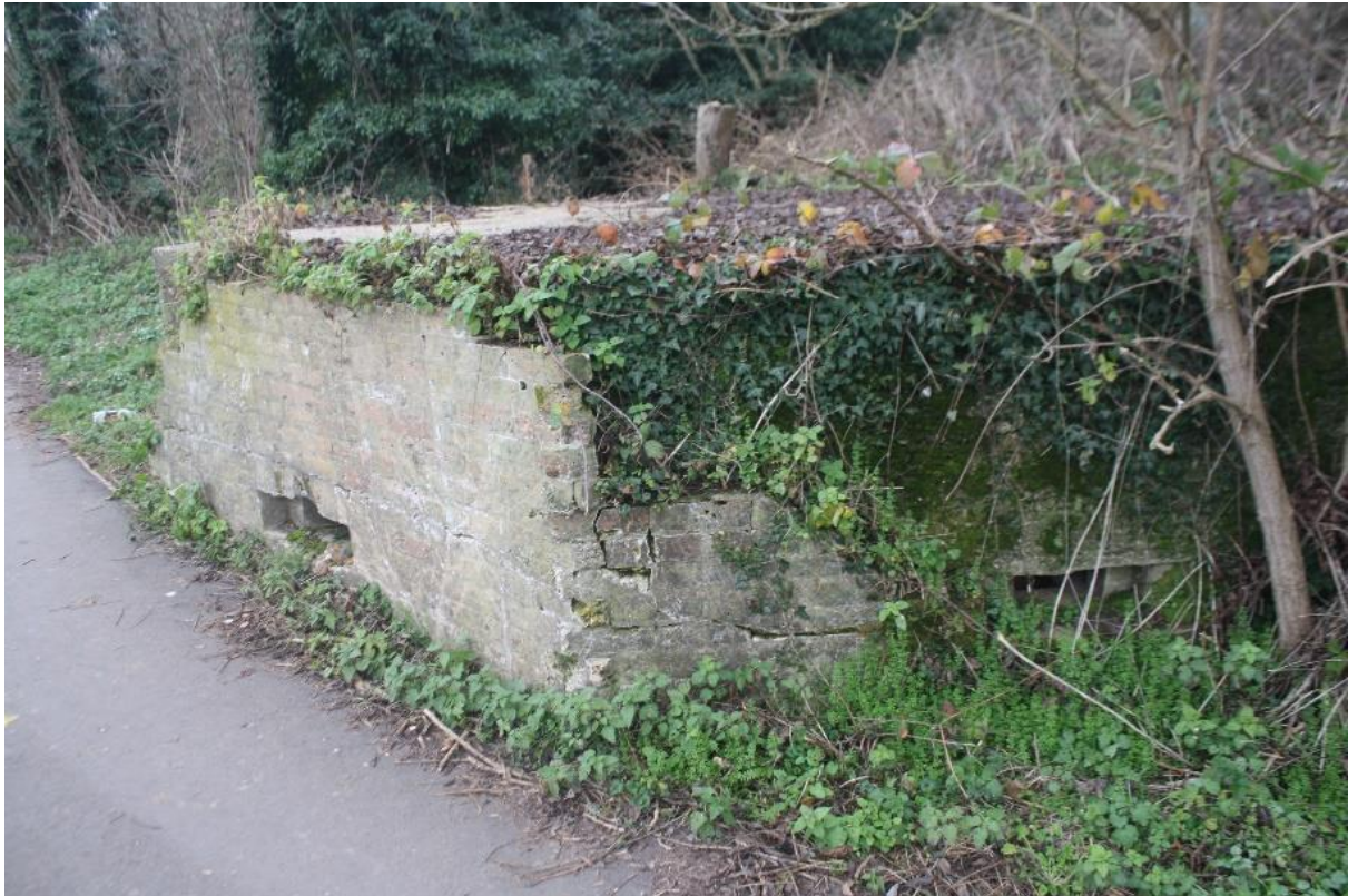
Recently exposed Type 24 pillbox by the Medway at East Farleigh
