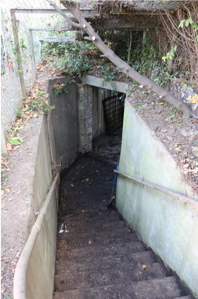
The entrance steps to the MGS shelter after clearance in October 2018
