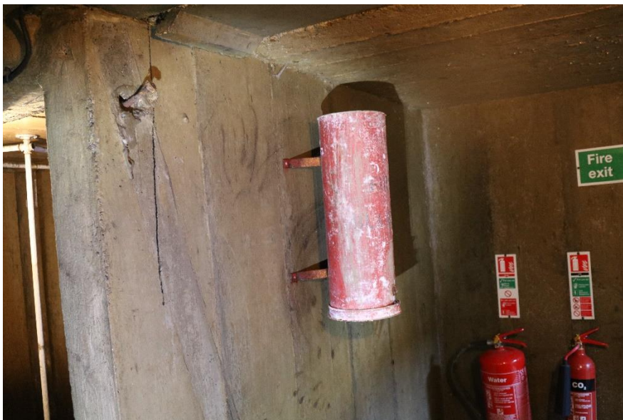
Original fire blanket container in the MGS shelter
