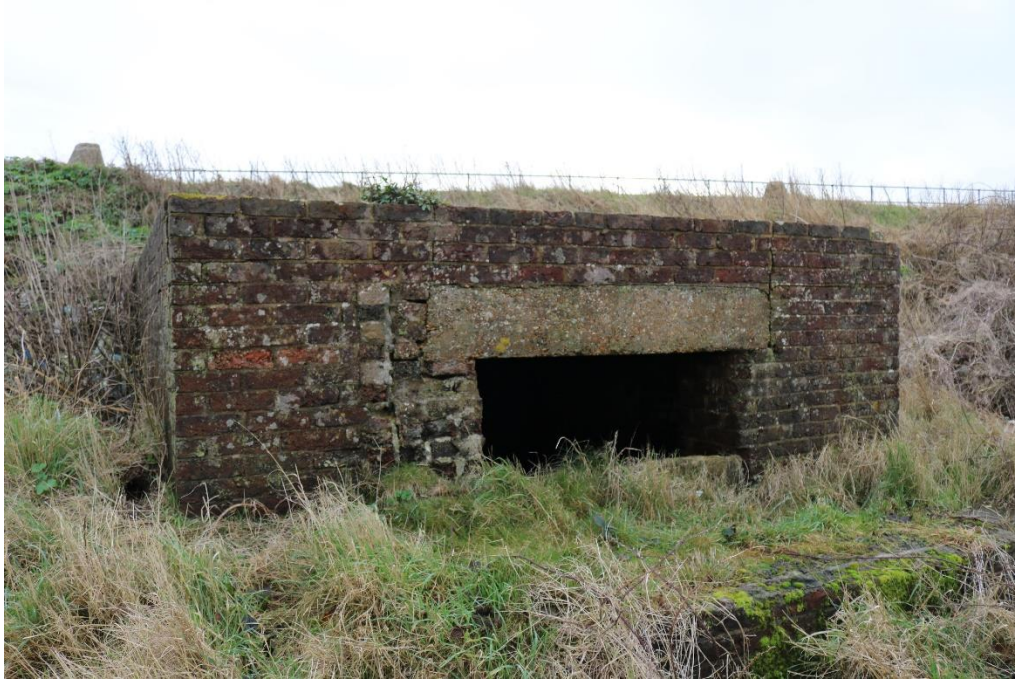
One of the Fougasse structures at Camber (rear view)
