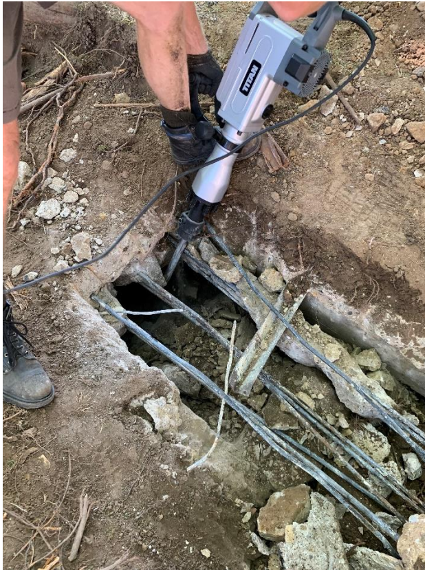
The electric breaker gradually exposing the entrance tunnel
