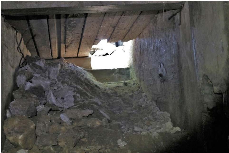
Inside view of the exposed entrance
