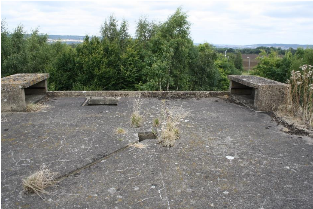
Bofors gun platform. Note the ammunition lockers. The void in the photo was for an external ladder.
