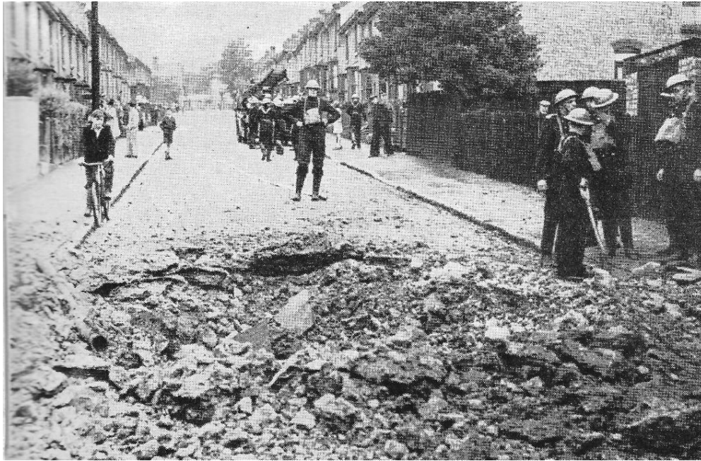
Bomb damage in Charlton Street, Maidstone. September 1940
