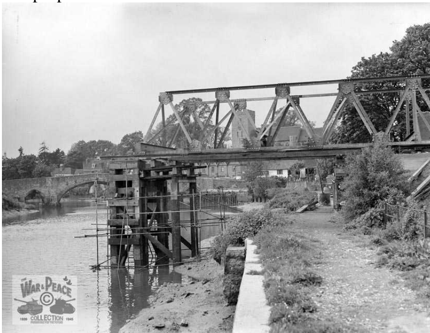
The Callender-Hamilton bridge under construction at Aylesford (War & Peace Collection)
