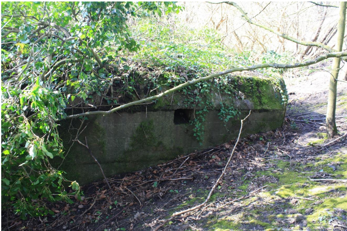
Type 28A pillbox near Teston Bridge
