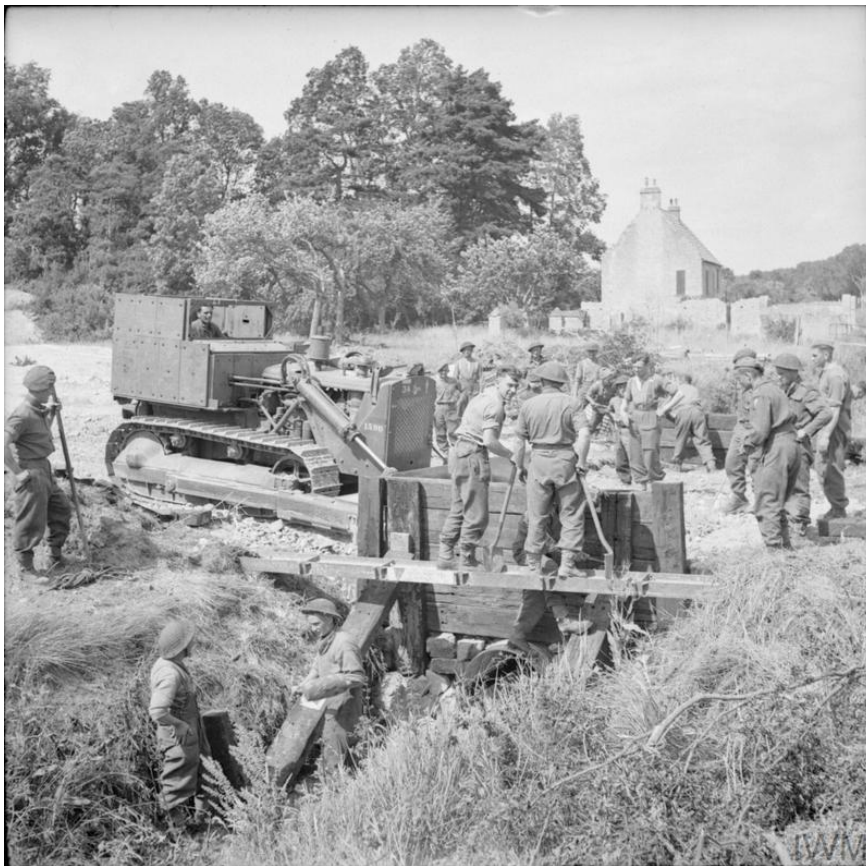
Royal Engineers angle dozer at work © IWM (B 6177)
