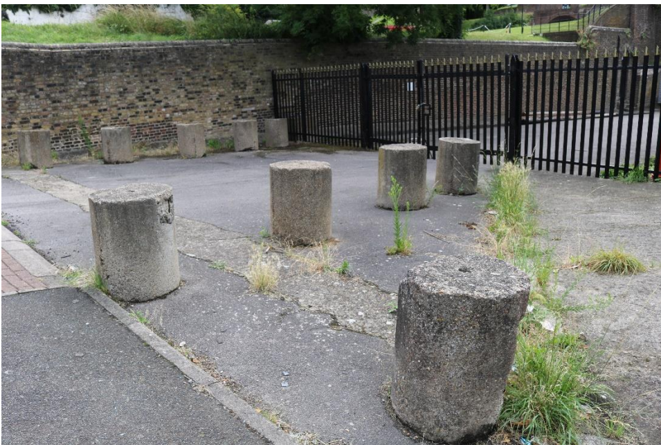
Movable 'Cylinder' obstacles at Fort Amherst, Chatham
