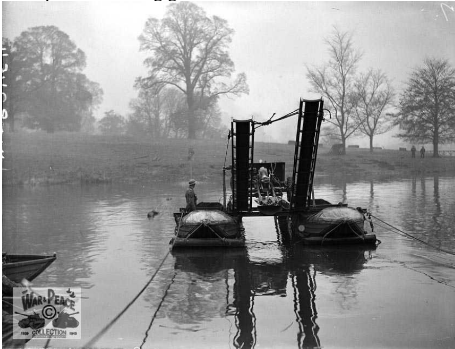
Royal Engineers ferrying a 25-pounder field gun across the lake at Mote Park (War & Peace Collection)
