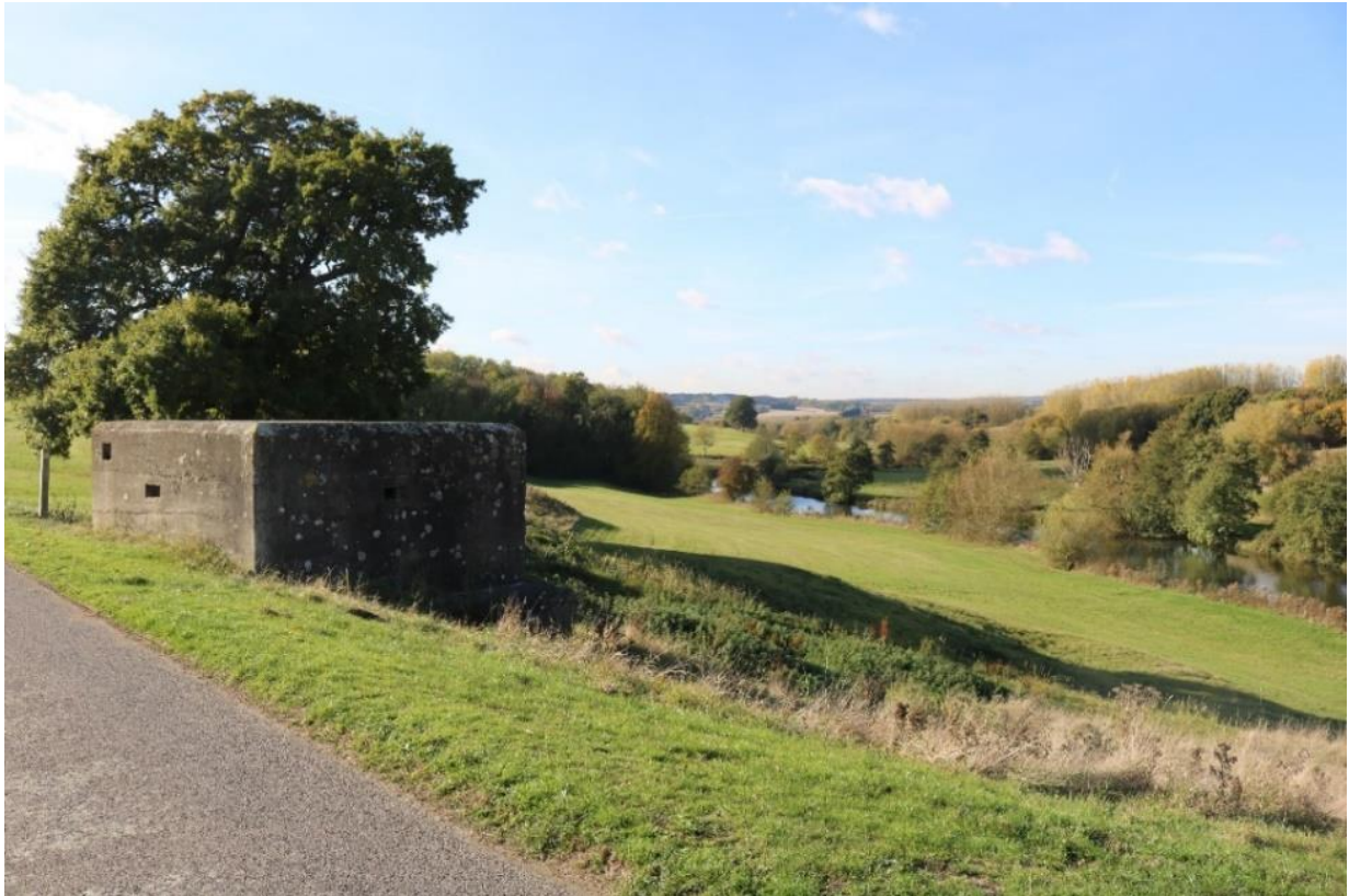
A shell-proofed machine-gun pillbox overlooking the Medway at Teston
