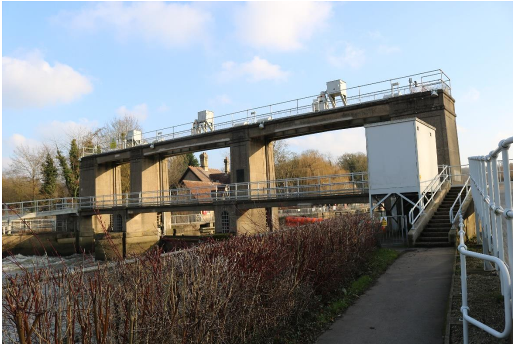
The sluice gates at Allington Lock
