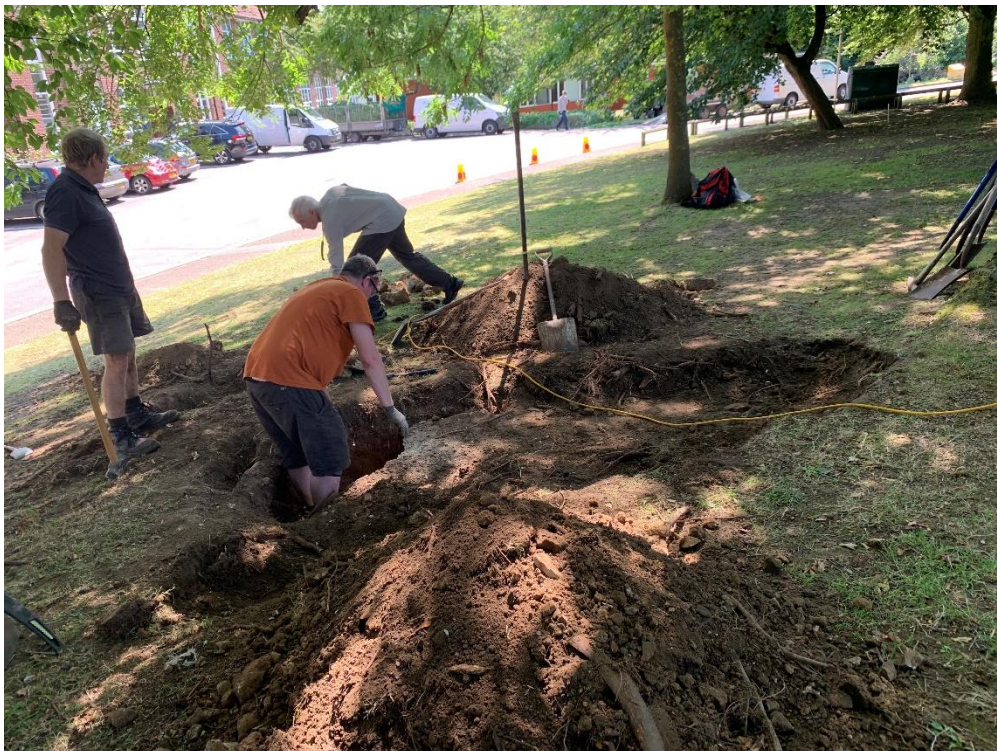
Some of the KURG team digging out the MGGS shelter entrance
