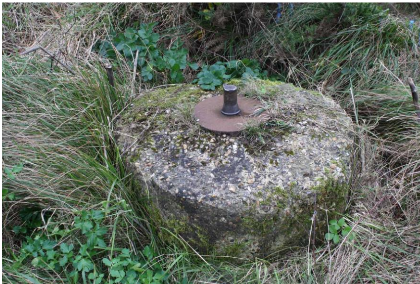
A surviving spigot mortar concrete pedestal at the Citadel Battery, Dover
