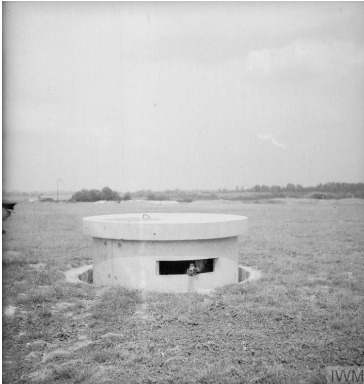
The turret of a Pickett-Hamilton Retractable Fort, fully raised and manned by a bren-gun team of the Coldstream Guards, taken on a fighter airfield in Southern England. © IWM (CH 17890)
