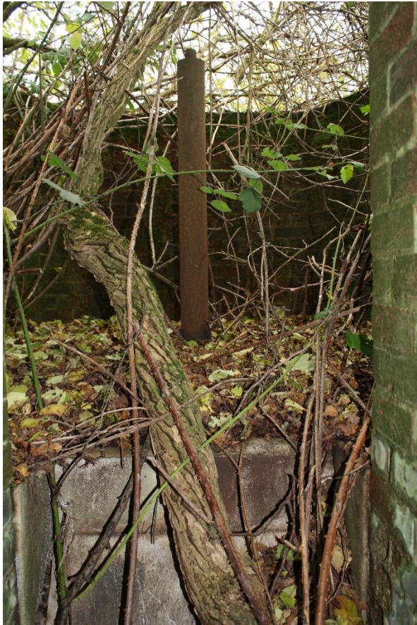
Internal view of the LAA gun well showing the gun mounting
