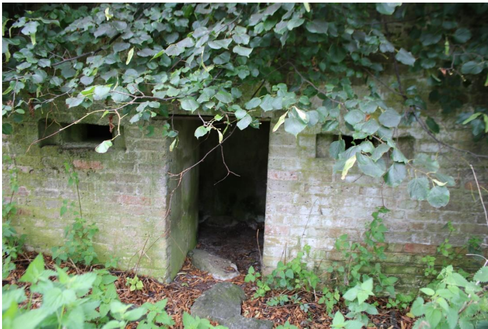
The rear wall of a Type FW3/24 at Teston showing the entrance
