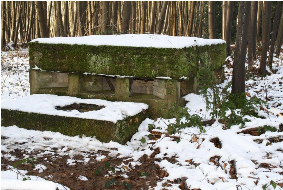
Observation room and emergency escape hatch
