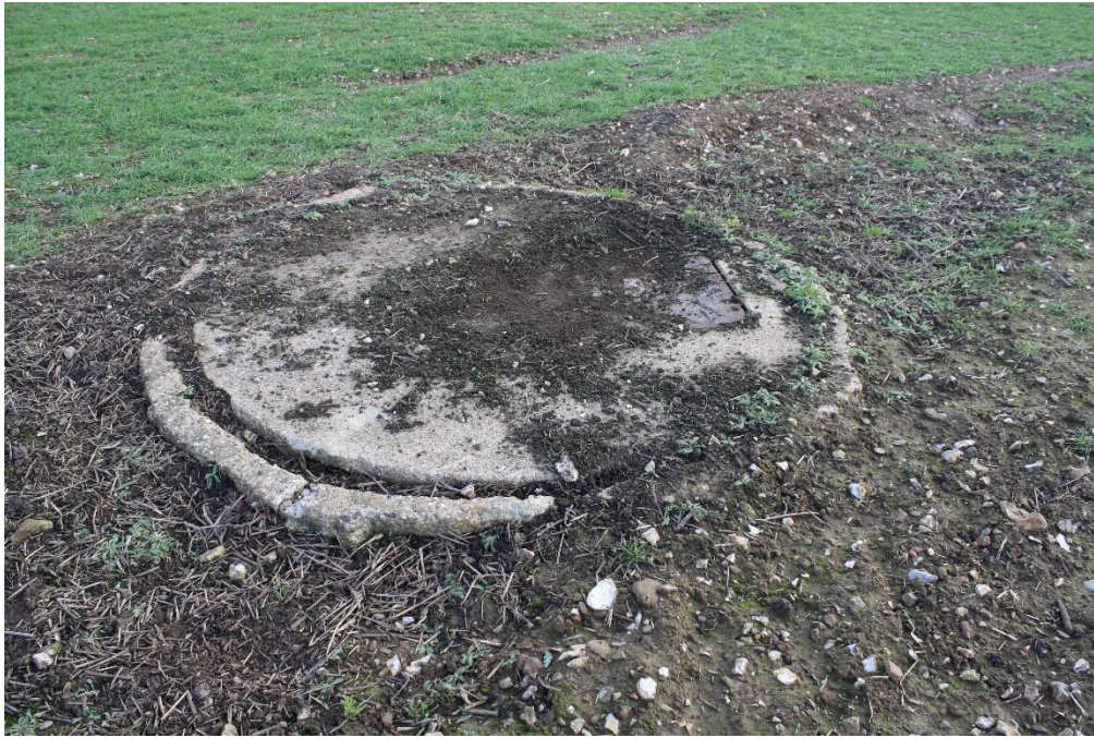
A fully retracted Pickett-Hamilton Fort at Detling, The access hatch off-centre to the right
