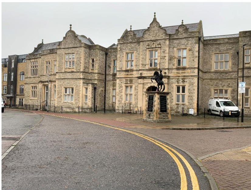
The former Kent County Ophthalmic Hospital in Church Street
