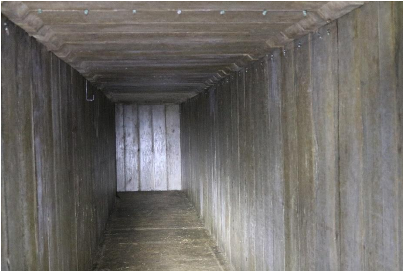
Internal view of one of the shelter's 'classrooms'
