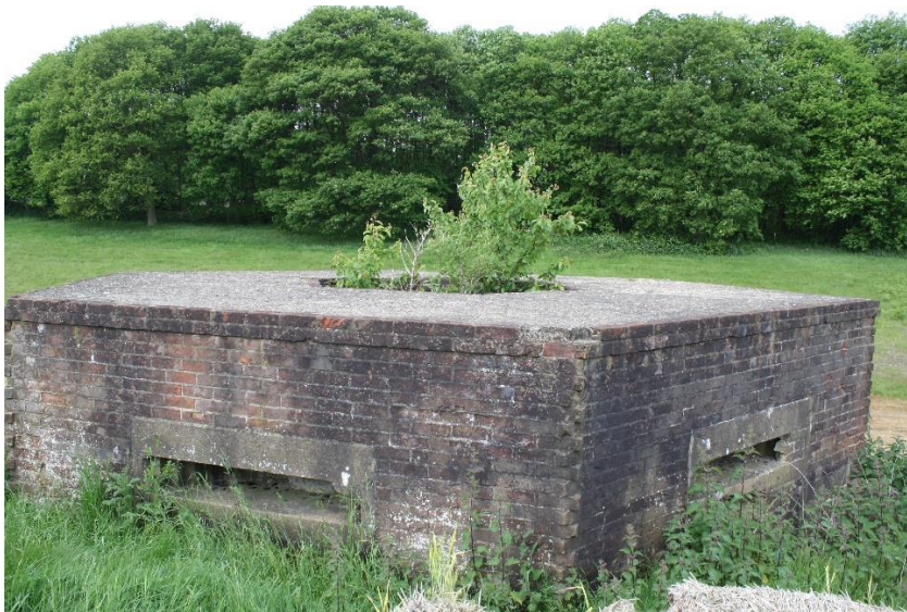
Bullet-proof version. Note the vegetation growing out of the central LAA gun well
