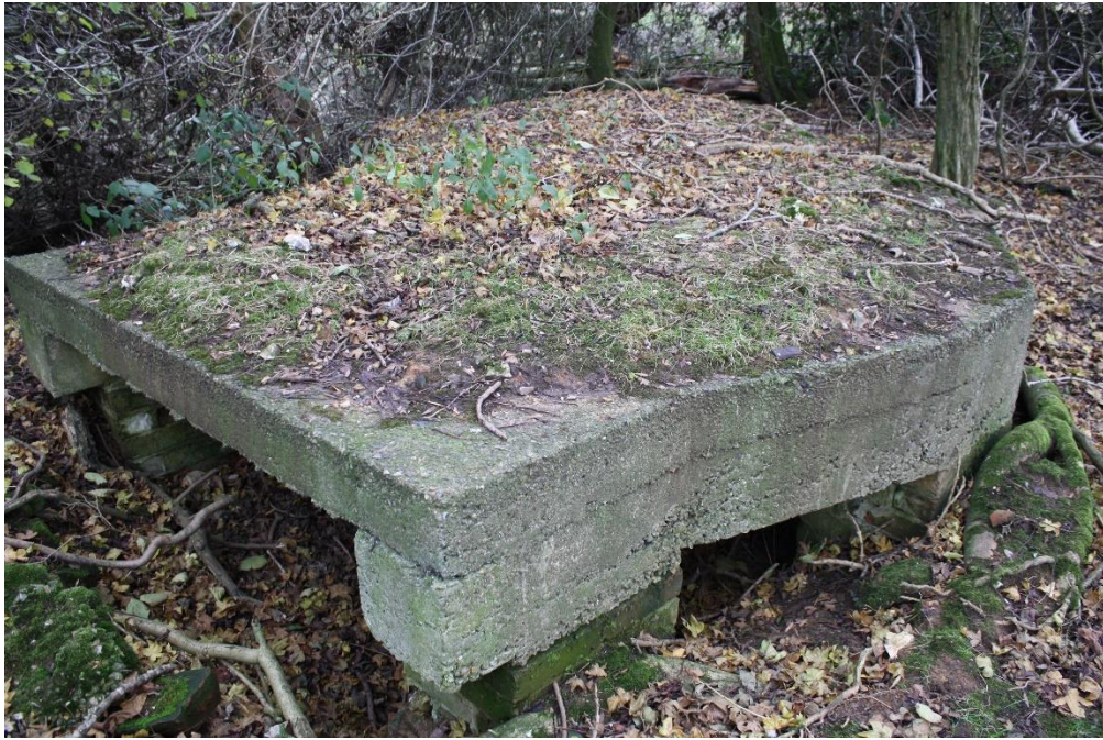
The distinctive 'seagull wing' shape of the roof
