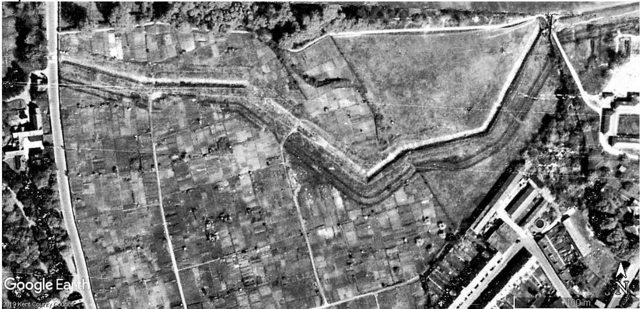
The anti-tank ditch and obstacle line running across Allotment Gardens from the A229 Chatham Road
