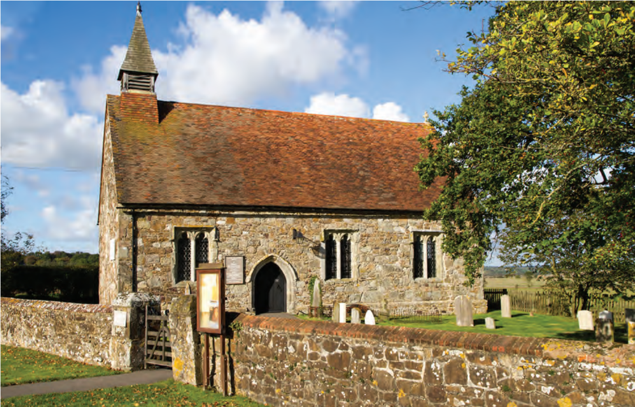
The church from the south, showing three of the windows salvaged from the Elizabethan St Mary's. ©Stuart Kirk
