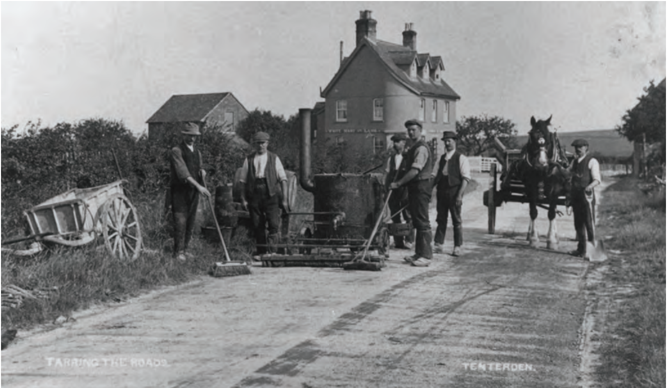
Resurfacing the junction of the two former turnpike roads at Reading Street c. 1925. 'The White Hart and Lamb' inn is in the background. Turn left here for Appledore and New Romney; straight ahead for Wittersham and Rye.
